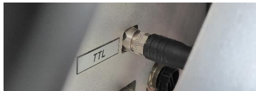
Connected “TTL” cable.
