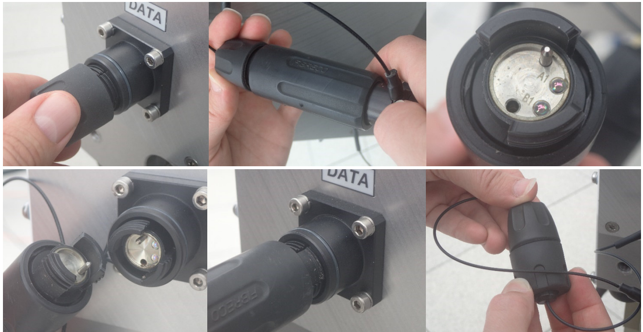
Connecting the fiber optics data cable.
