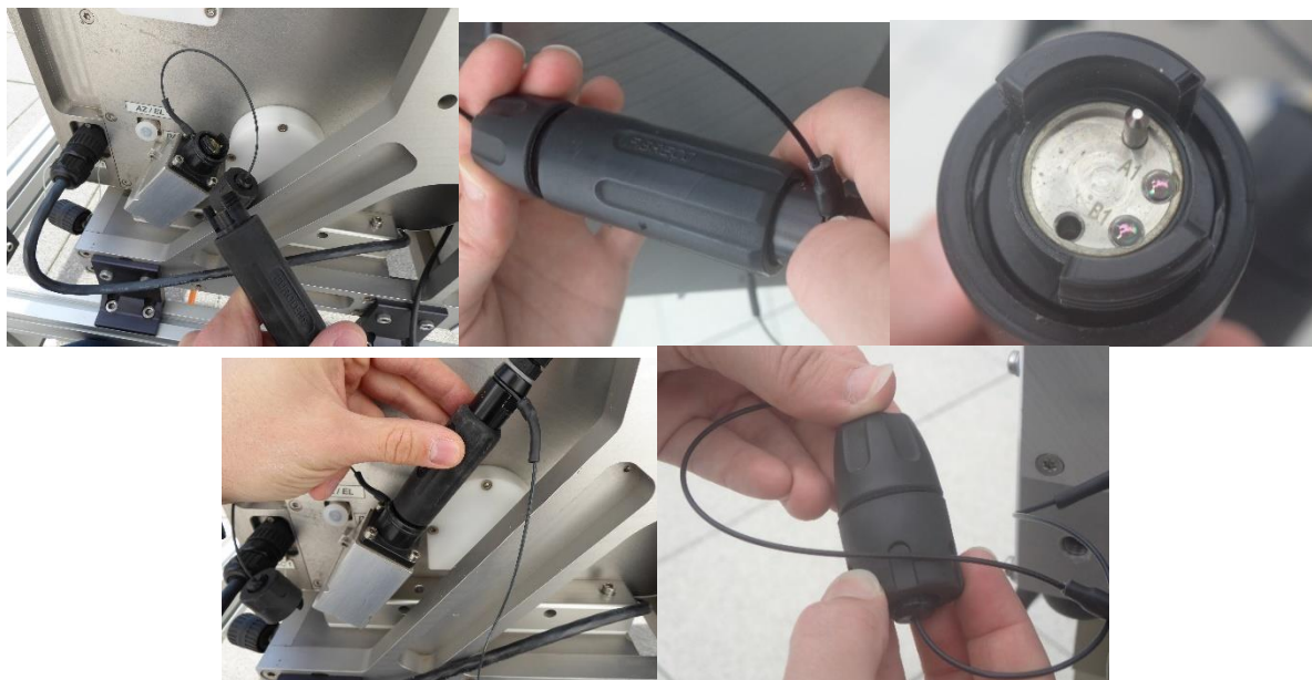
Connecting the fiber optics data cable.
