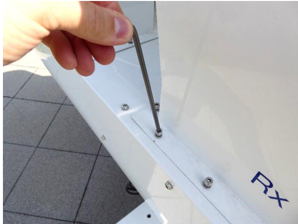
Use Allen key to fasten the air guides.
