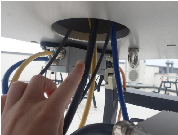
Fig.2.5.8: Pulling back the cables to adjust the cable lengths.
