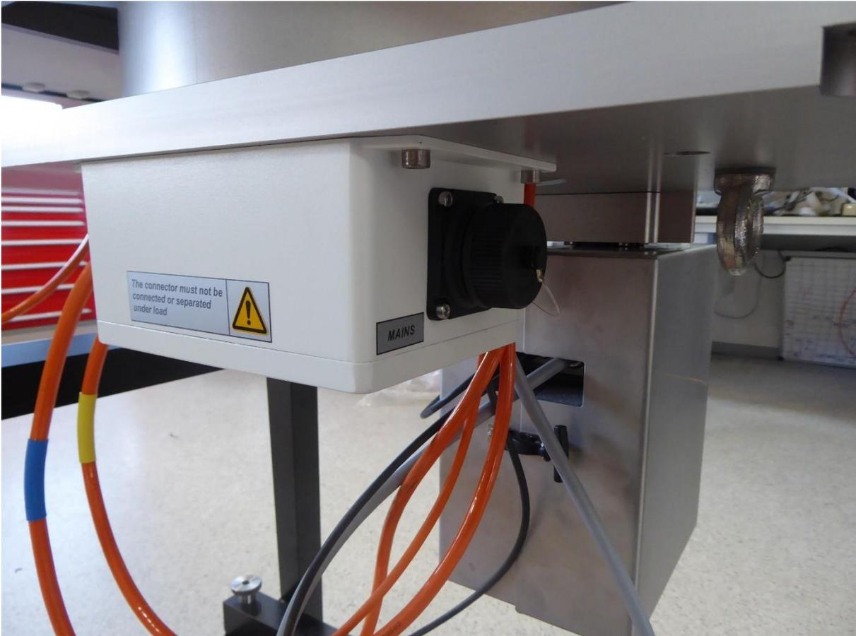
**(Fig.2.5.46): attach the knurled nuts to tight the frame**
