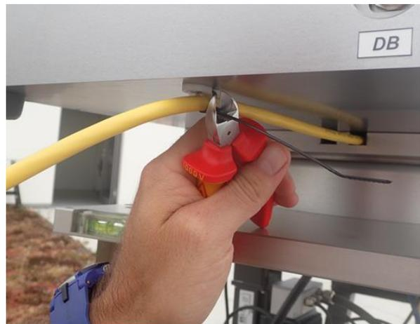
**Fig.2.5.32: Fixing AC2 cable on radiometer bottom plate and cutting the cable tie.**
