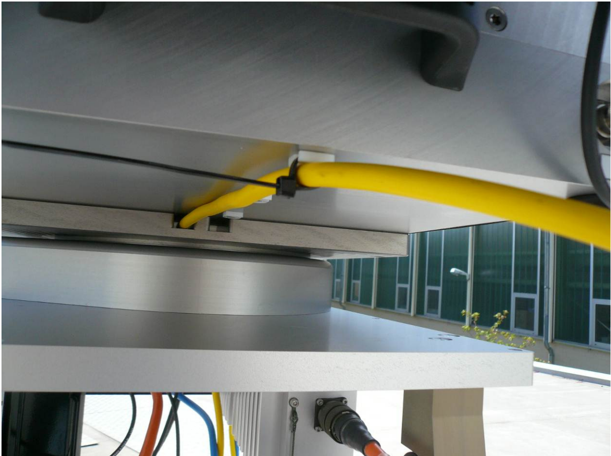
Fig.2.6.8: Fixing AC2 cable on radiometer bottom plate.
