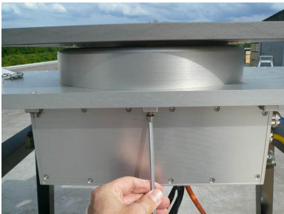
Fig.2.4.5: Mounting the azimuth drive power supply.
