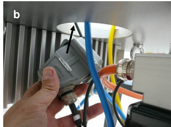
Fig.2.4.10: Feeding AC1, AC2, DATA/AZ and fibre optics data cable through centre hole.
