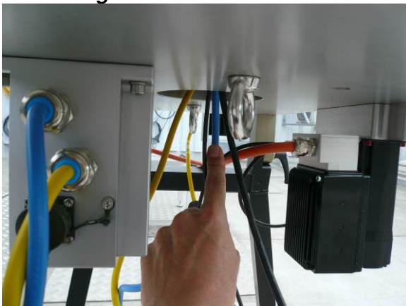
Fig.2.5.9: Pulling back the cables to adjust the cable lengths.
