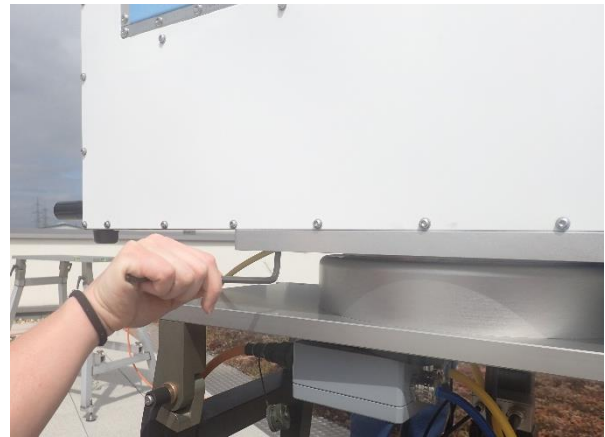
Fig.2.5.3: Use Allen key to fasten the box with four M8 screws.
