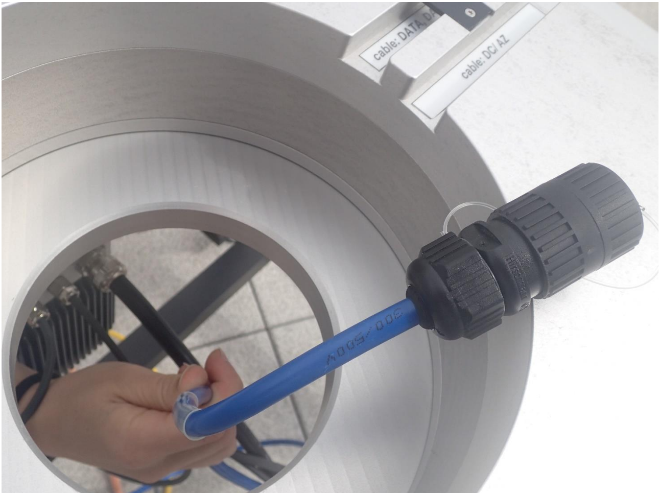
Fig. 2.4.7. Feeding AC1 cable through center hole. Do the same for AC2, DATA/AZ, fiber optics data and DC/AZ cable.
