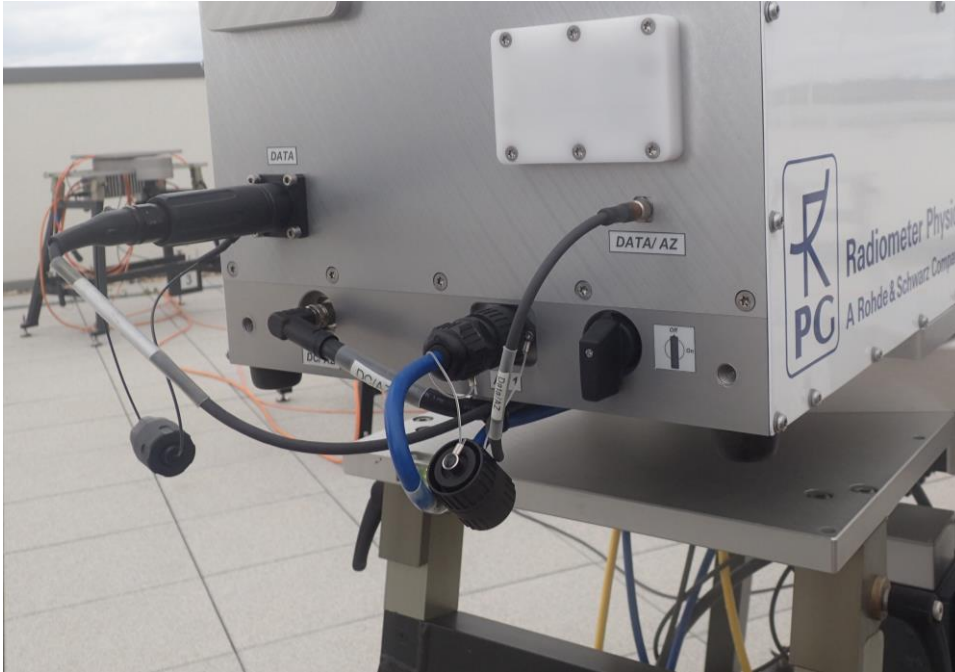
Fig.2.5.8: All cables connected to the radiometer.
